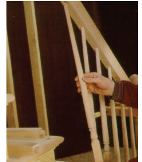
Rake rails on stair are drilled for easy baluster insertion, up into rail and down into tread.
