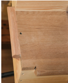
Stair is notched for post.
