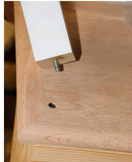
Treads are drilled for balusters, and inserts are installed.
