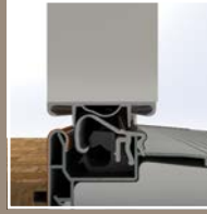
Cap rises to engage door bottom
